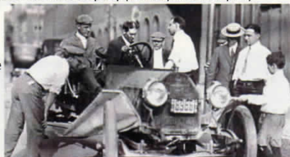
Charles F. Kettering (at the wheel) and Bill Chryst (in passenger seat) test the Delco Self-Starter System invented by Kettering in Dayton
